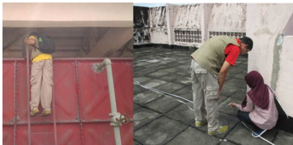
Volunteers conducting the Building Condition Assessment.
