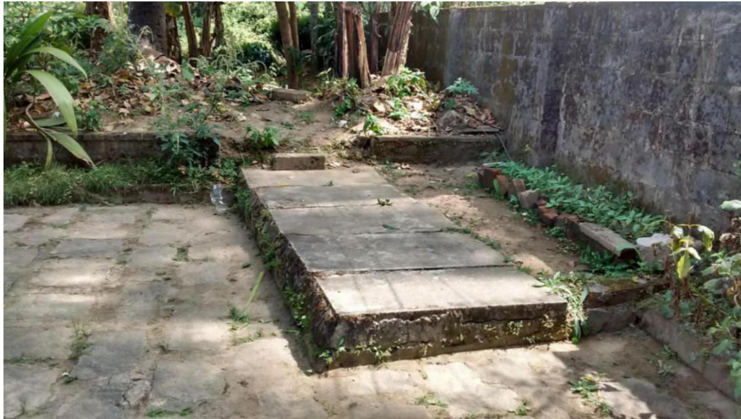
Figure 2: A three chambered septic tank connected to soak pit of a HH (Source: Anil/CSE, 2017)
