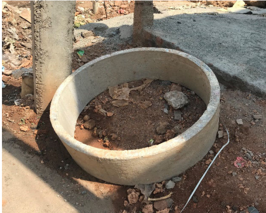
Figure 10: A pre-fabricated concrete ring found near an under-construction house (Harsh/GIZ,2019)
