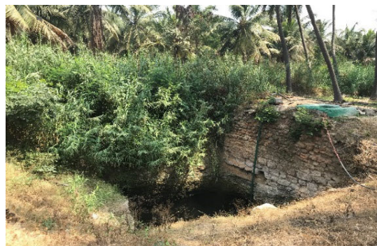
Figure 6: Open well comprising of inflow sewage of Ondipudur STP (Kripa/Eawag,2019)
