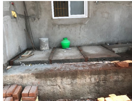
Figure 8: Under-construction Rectangular Fully Lined Tank (FLT) sealed (Harsh/GIZ,2019)
