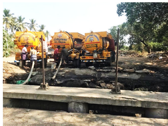
Figure 11: Septage Decanting Point near Ukkadam STP (Harsh/GIZ,219)
