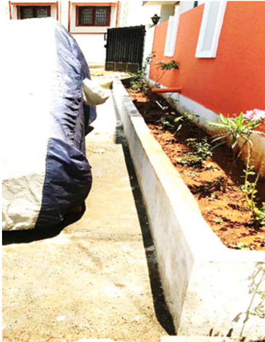
Figure 2: Recharge beds used for greywater discharge (Harsh/GIZ,2019)
