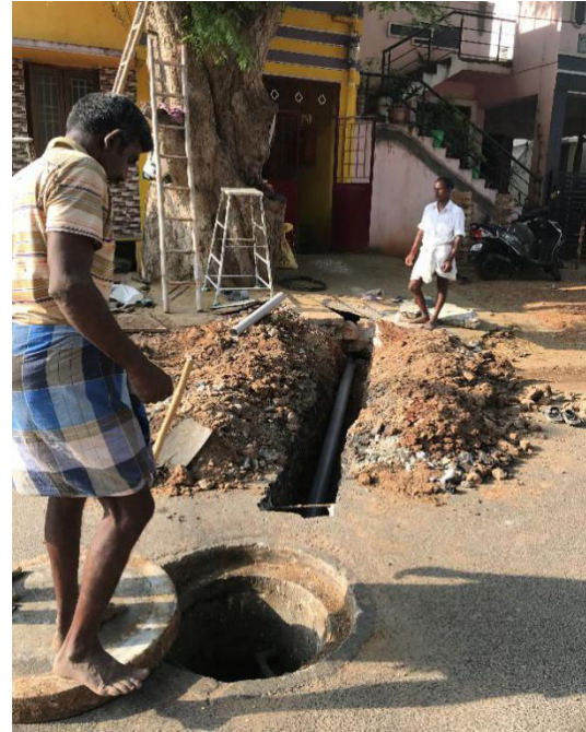
Figure 3: Household sewer connection in progress in ward 11 (Harsh/GIZ,2019)
