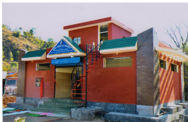
An example of: PT constructed using Cement blocks available locally
