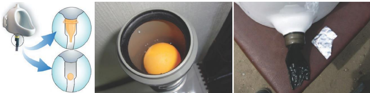
Figure 20: Low-cost odour control measures for waterless urinals or UD toilets (WECF, 2015, p. 34, adapted).
