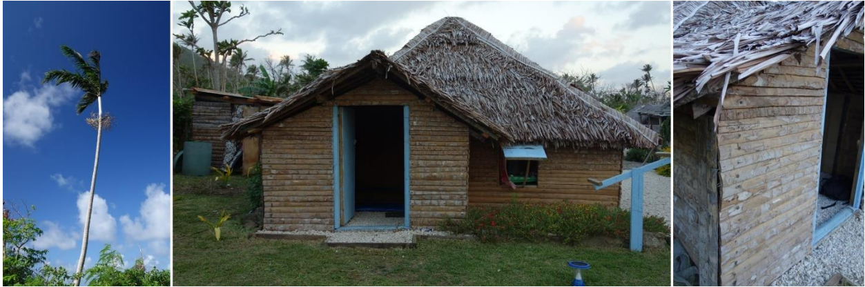
Figure 31: Coconut palm planks used as wall covering for traditional house on Emae, Vanuatu.
