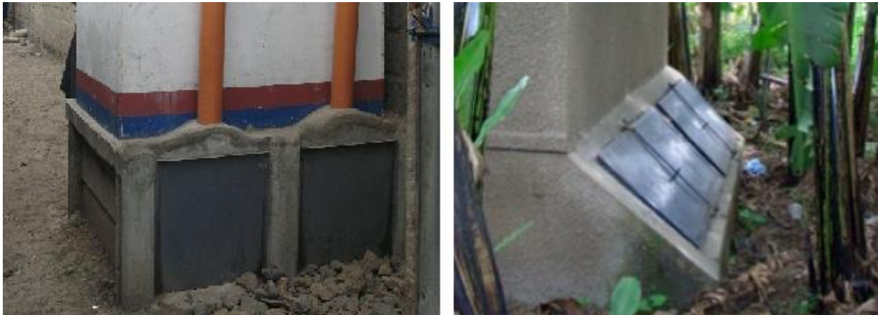
Figure 9: Straight vault doors of UDDT (left) (GTZ Ecosan, 2019, adapted; inclined vault doors of UDDT (right) Winberg & Otterpohl (2016, p.1227, adapted).
