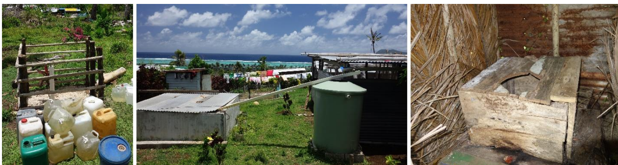
Figure 22: Springwater-fed tap (left); Rainwater harvesting incl. a ferrocement and a polyethylene tank (centre); bush toilet (right).
