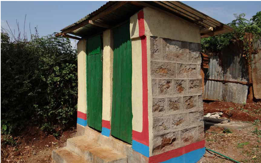
Picture 3: Toilets constructed under the UBSUP programme, Kenya
