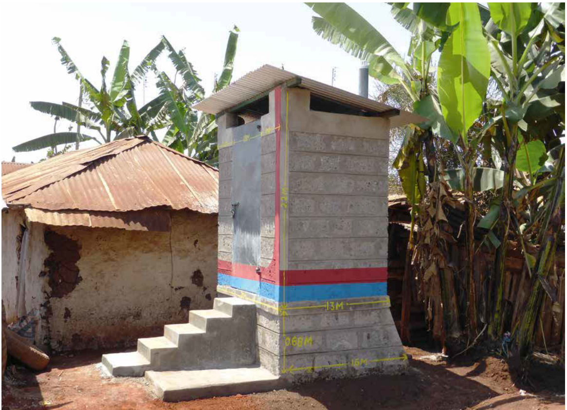
Picture 5: Toilet in Embu, constructed as part of the UBSUP programme, Kenya
