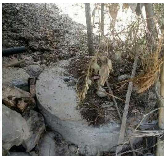
Figure 2: Pit with semi-permeable walls and open bottom (HHs survey, 2019).
