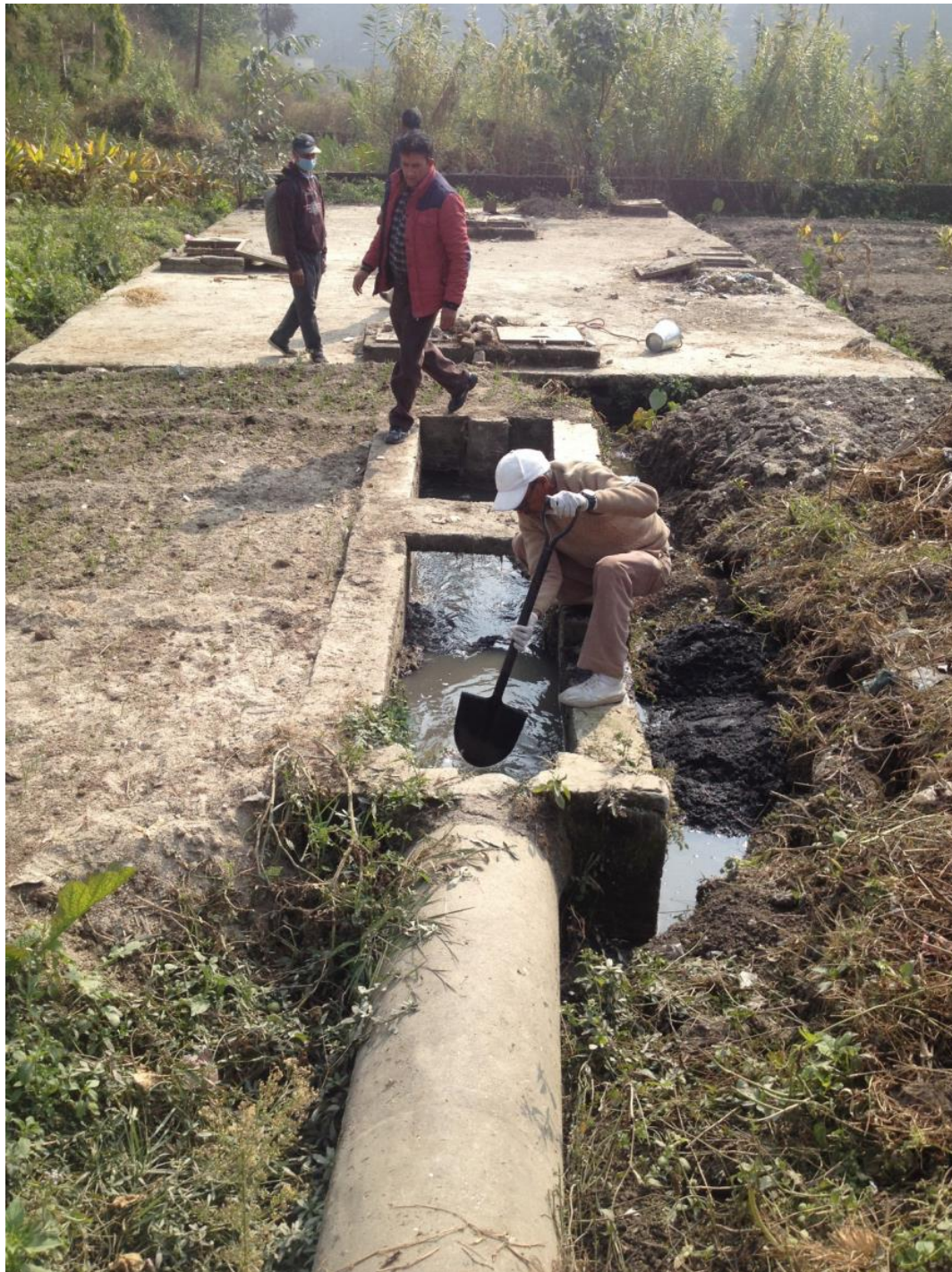
Figure 4: Decentralized Wastewater Treatment System.
