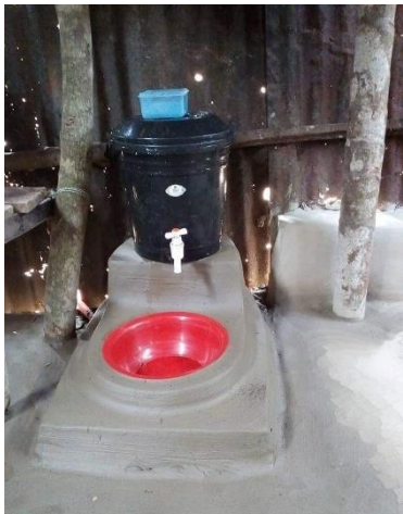
Bucket with tap, installed inside the kitchen along with plastic bowl for basin
