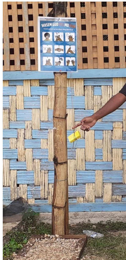
Figure 16: Completed bamboo handwashing station. Credit: World Vision International - Vanuatu
