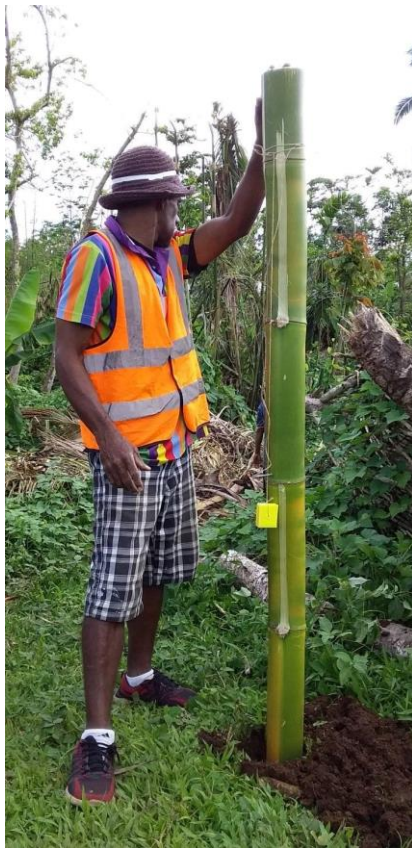
Figure 15: New bamboo handwashing station being inserted into the ground. Credit: World Vision International - Vanuatu
