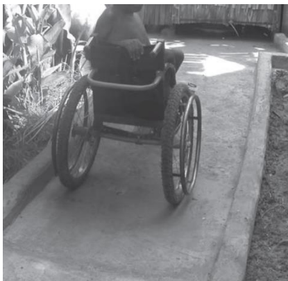
Figure 2: Wide concrete path with raised edges. Credit: Jones and Reed (2005)
