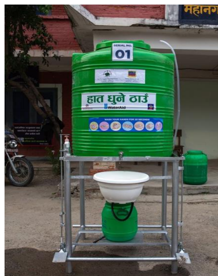
Figure 18: pedal-operated handwashing station with large tank. Credit: WaterAid Nepal
