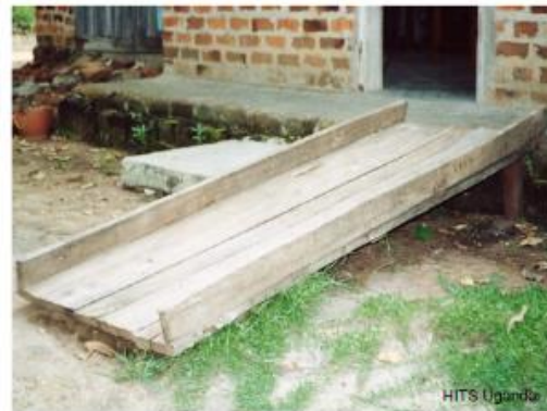
Figure 5: A temporary/movable wooden ramp. Credit: Jones and Wilbur (2014)
