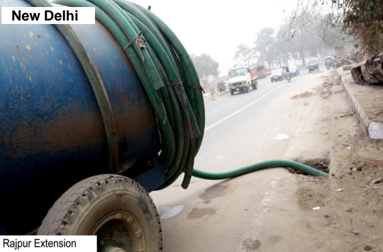
Septage disposal into storm water drain
