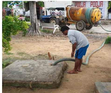
Figure 7: Emptying of ST by Private vacuum tractor (Source: Niharika/CSE, 2020)
