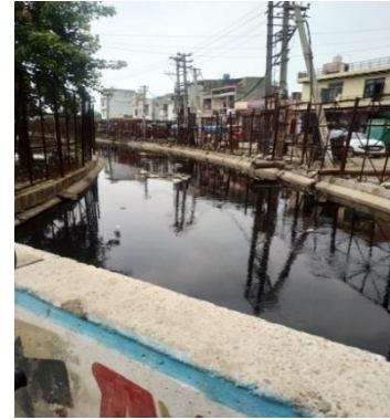
Figure 2: Untreated wastewater in Canal is flowing through the city (Source: Niharika/CSE, 2020)
