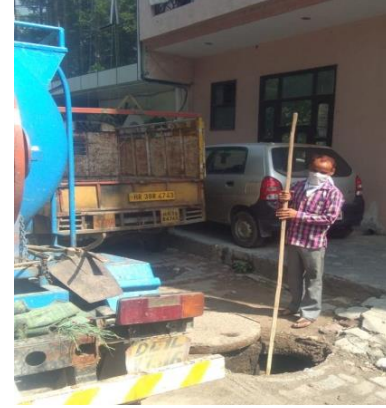
Figure 9: Sewer cleaning in ward no. 12 (Niharika/CSE, 2020)
