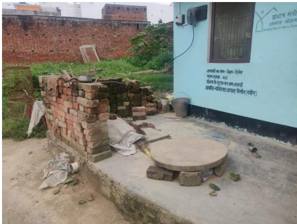
Figure 3: Septic Tank constructed under PMAY
