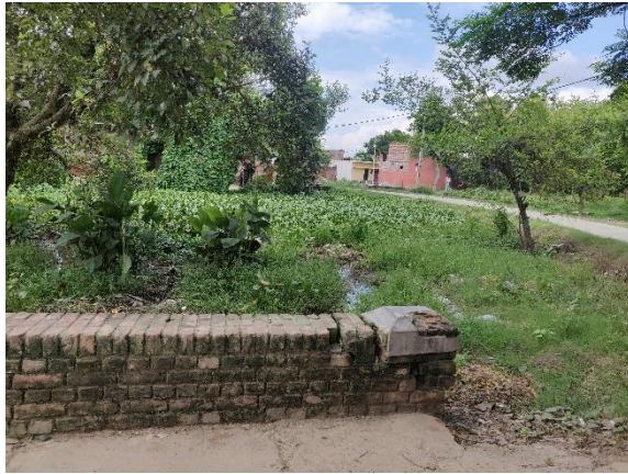
Figure 6: Drain in Ward 5
