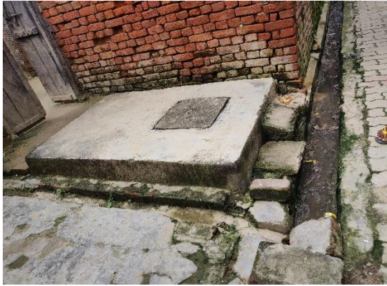
Figure 1: Overflowing containment system (Nida, CSE, 2020)
