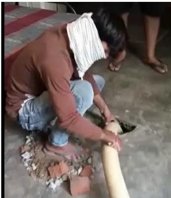
Figure 5 : Emptying in process by mechanical means (Harsh/CSE/2020)
