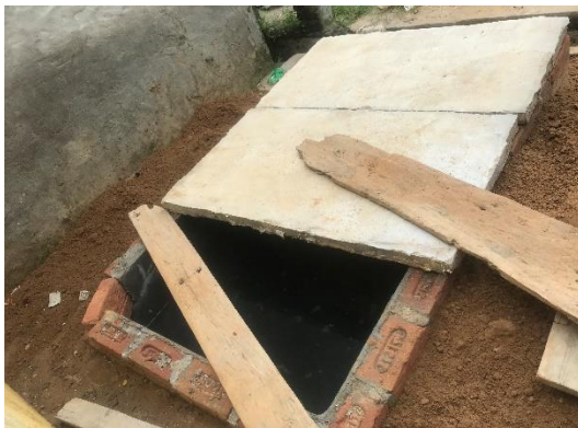
Figure 3: A septic tank under construction. (Harsh/CSE/2020)
