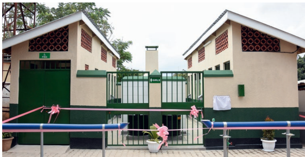
Figure 1: Toilet block with PWD cubicle in the girls' wing at St Peter's Primary School Nsambya, with WASHaLOT 3.0 group handwashing facilities in front.
