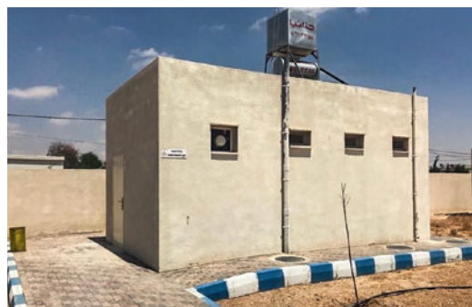
Figure 8: Accessible toilets at Salah Eddin Mosque, Mafrqa.
