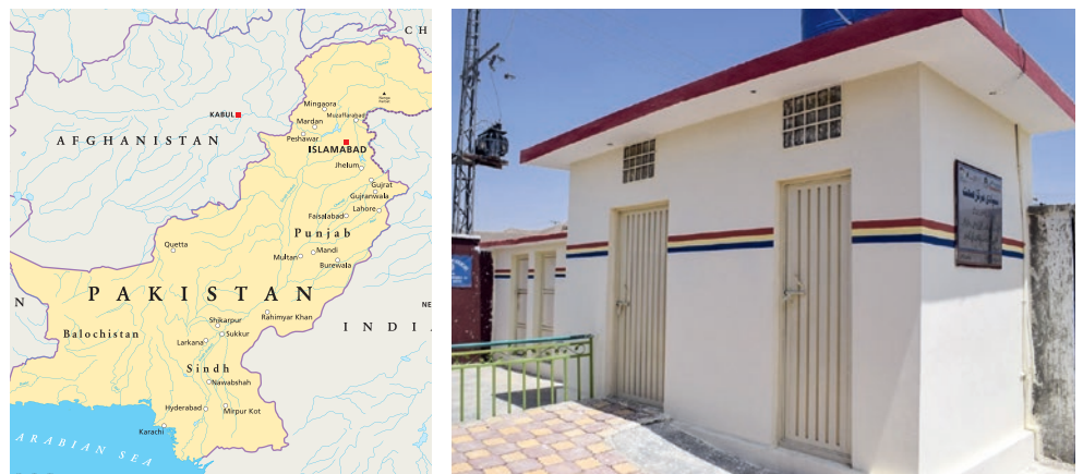
Figure 4: New toilet facilities at a basic health unit in Quetta district, Balochistan, Pakistan.
