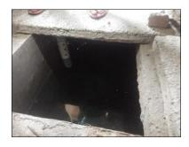
Figure 2: Septic tank connected to open drain
