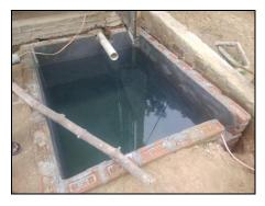
Figure 3 : under construction single chamber fully lined tank
