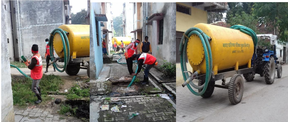
Figure 2: Mechanical emptying in process (on left) and tractor mounted vacuum tanker (on right) (Manish/CSE, 2020)
