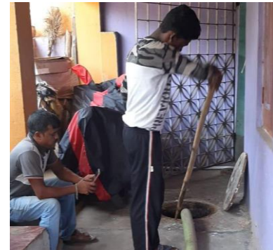
Fig 4: Emptying Onsite Sanitation System by Vacuum Tanker (Source: CSE,2020)
