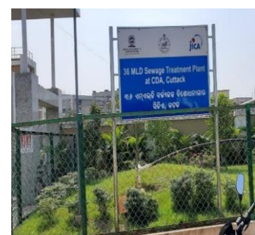
Fig 1: Sewage Treatment Plant (Source: CSE, 2020)
