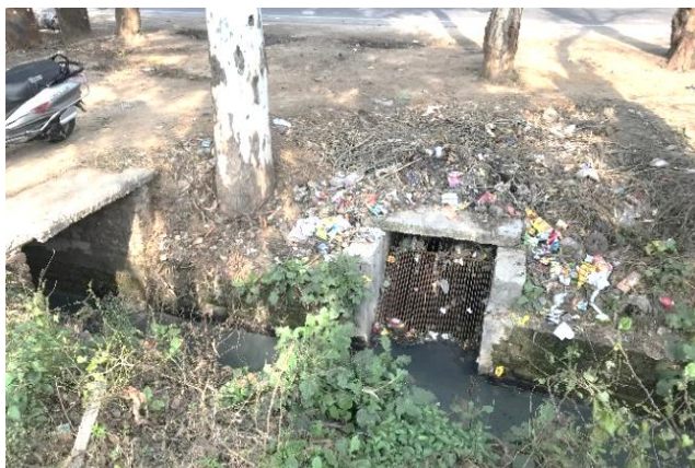
Figure 1: Open Drain tapped at Barrage Road. (Harsh/CSE, 2020)
