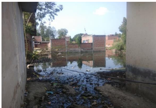
Open drain ending at open ground
