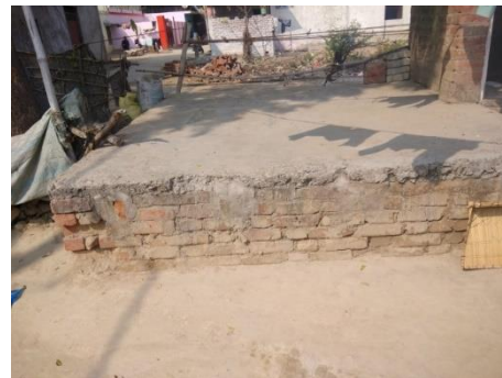
Fully lined tank
