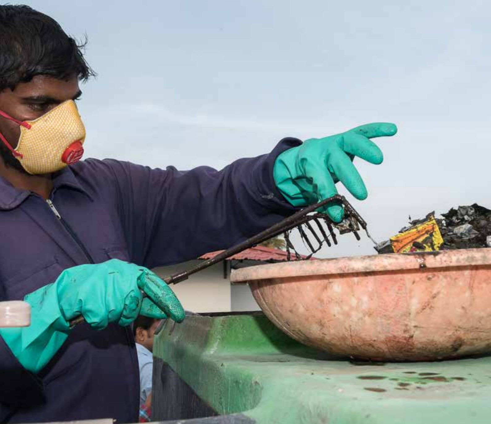
Figure 2 - Devanahalli FSTP operator, Mr. Raju performing regular cleaning operations of the feeding tank.
