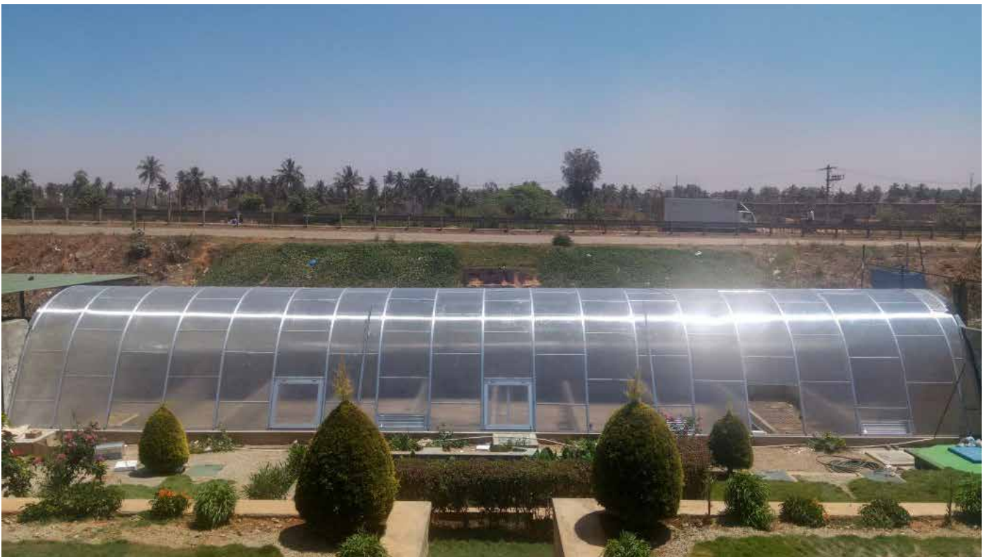
Figure 10 - Green house solar drier roof arrangement over the unplanted sludge drying beds for enhanced moisture removal
