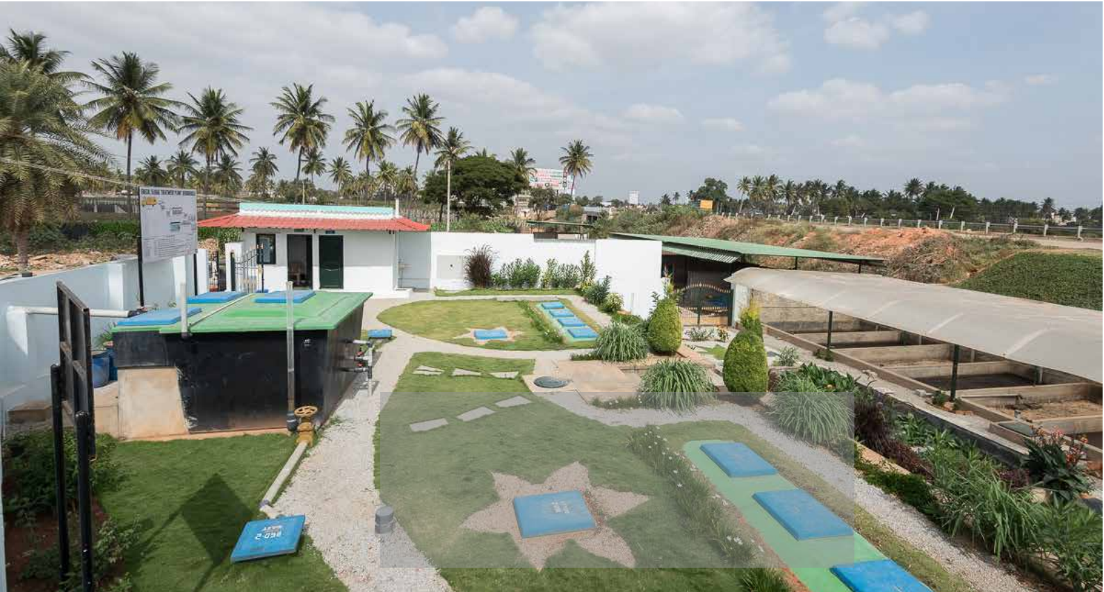
Figure 7 (Top) - Highlighted portion shows the original biogas digester and stabilisation tank that was replaced with a Stabilisation Reactor
