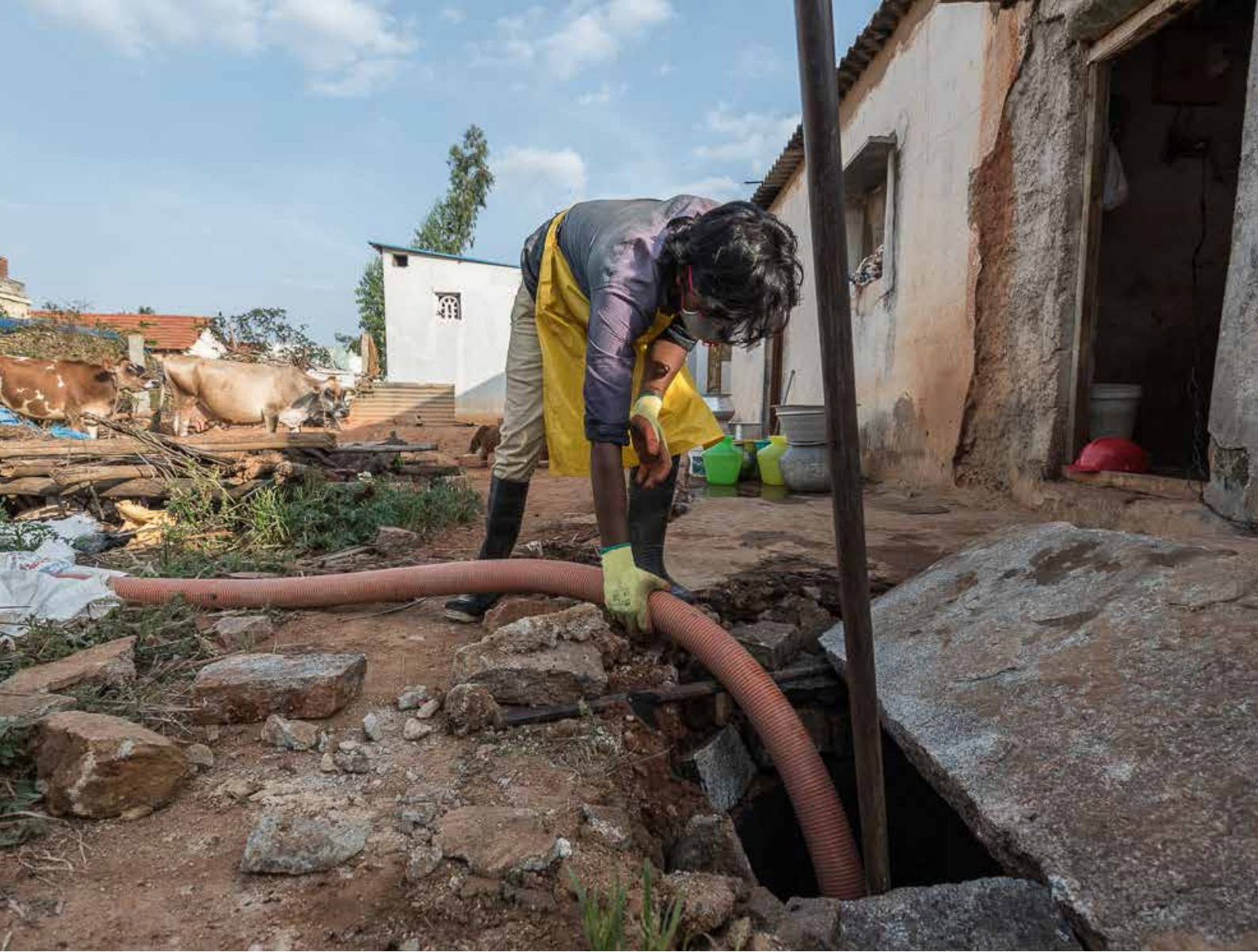
Figure 5 (Top) & 6 (Bottom) - Desludging of a pit in Devanahalli
