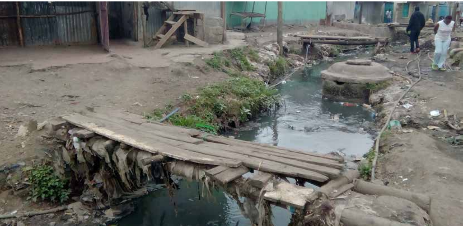
The main wastewater disposal tunnel in Zone 48.
