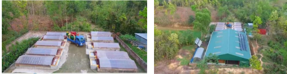
Figure 4: Sakhipur Faecal Sludge Treatment Plant (Co-compost plant).
