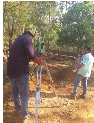
Survey work at site
