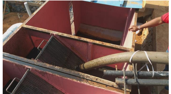
Septage Addition started on 10 th May 2019
