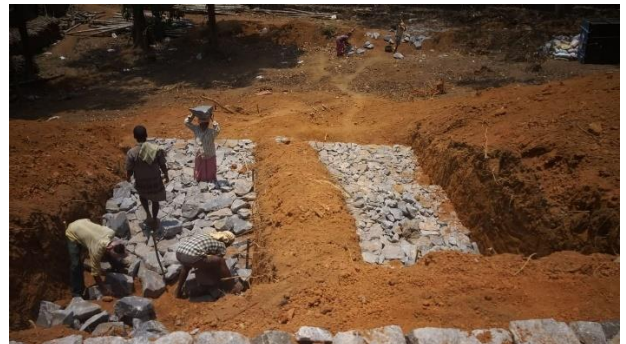
Rubble soling for anaerobic digester
