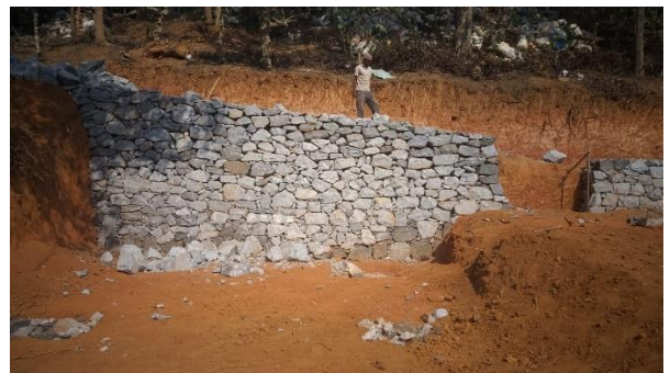
Retaining wall for cabin
