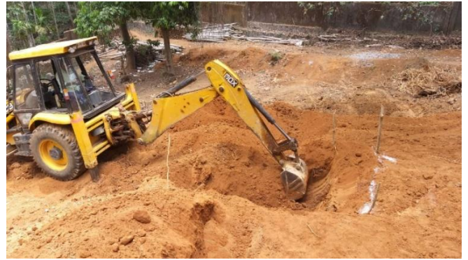
Excavation for storage tank
