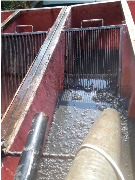
Septage Addition started on 10 th May 2019
