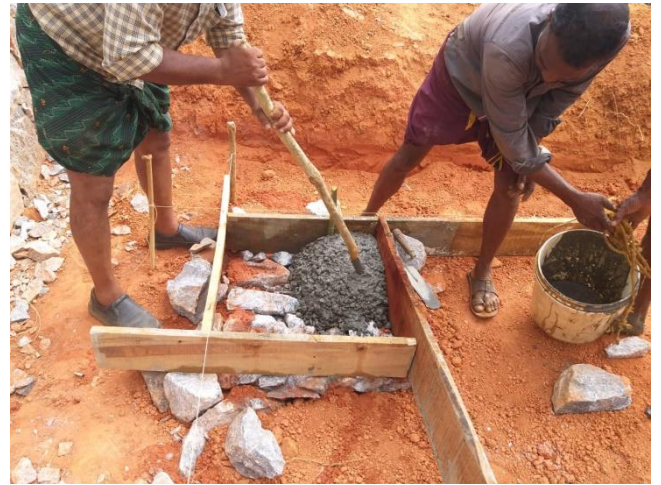
PCC work for cabin footing
