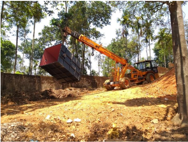
Unloading material with help of crane
