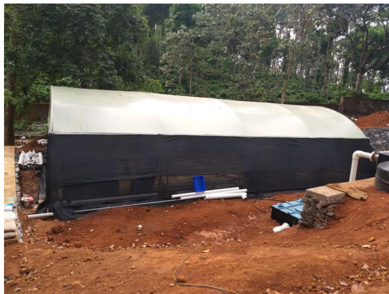
TBF Bed Containment Shed
