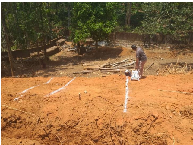
Site marking for anaerobic tank
