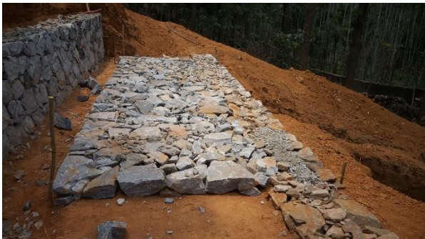
Rubble soling work for screen chamber tank
