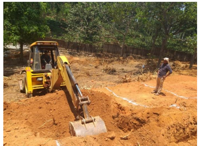
Excavation for anaerobic tank
