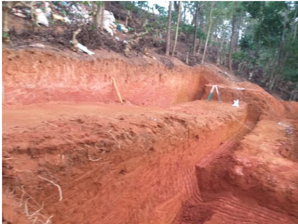
Site levelling after excavation for cabin
