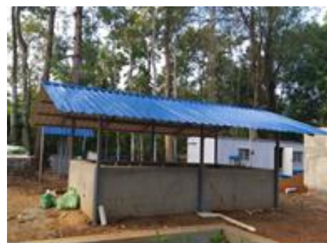
Shed for protection
