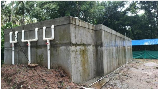
ASR Valve Arrangement
