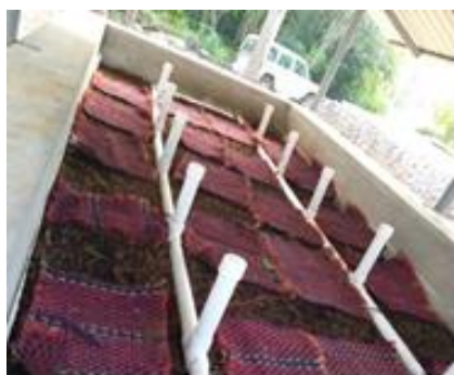
Distribution arrangement through the channels
