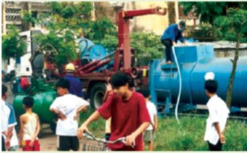
Intermediate storage tanks
