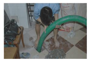
**Figure 3.13** A septic tank located below a house, requiring the floor to be broken for emptying or sampling, Hanoi, Vietnam (photo: Eawag).
