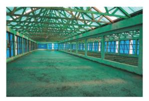
**Figure 4.2** Settling-thickening tanks at Lubigi FSTP in Kampala, Uganda (photo: Eawag).
