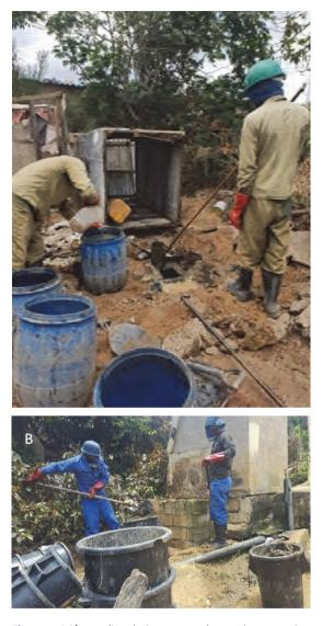
Figure 3.16 A) sampling during a manual emptying operation in Lusaka, Zambia, and B) Durban, South Africa (photos: Eawag).
