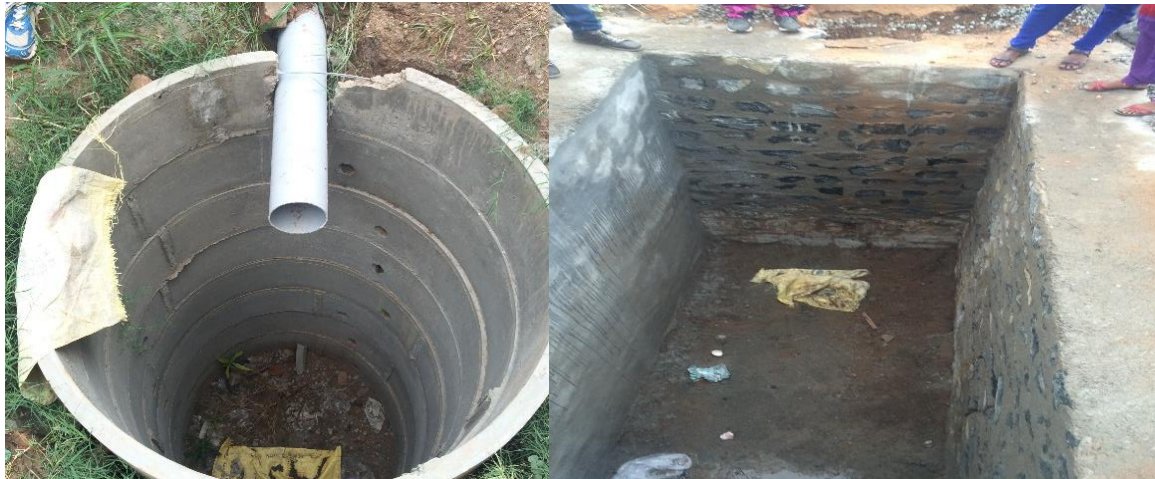
Figure 4.9: Containment structures in Town Panchayats
