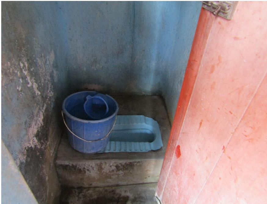
Figure 3.3: Community toilet showing small plinth area
