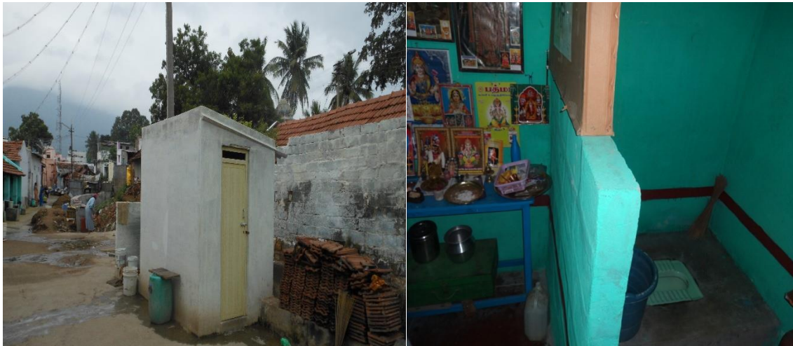
Figure 4.1: Household Toilets in Town Panchayats
