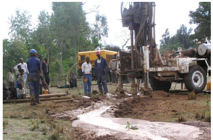
Figure 12: Drill rig with drilling fluid channel
