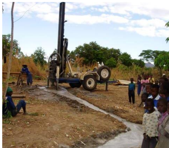
Figure 7: Controlling the discharging waters
