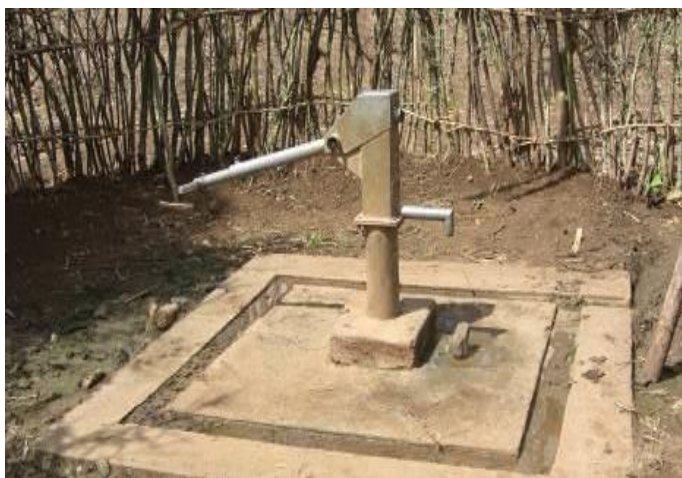
Figure 11: Rectangular pump platform (for wheelchair access)
