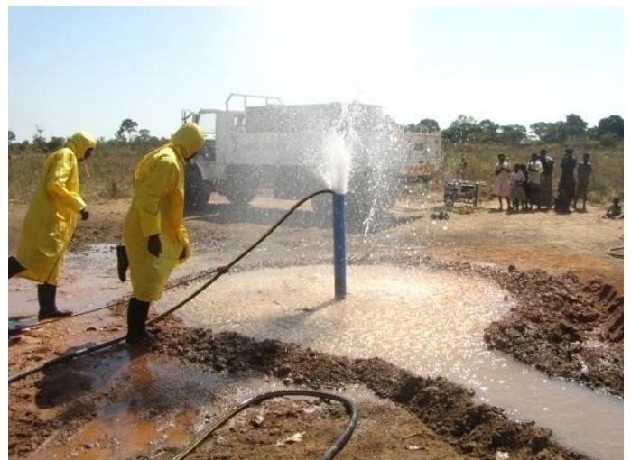
Figure 9: Cleaning the borehole with an air-jetting tool
