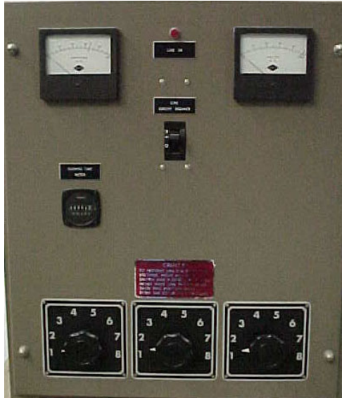
Figure 5 Tap Switch Voltage Control Rectifier
