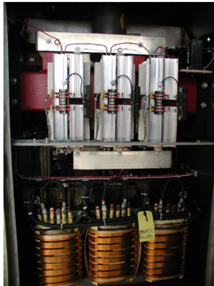
Figure 6 Typical SCR (Thyristor) Rectifier
