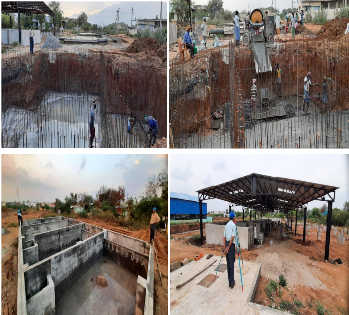
Figure 6. Under construction 30 KLD capacity FSTP at Srivilliputhur (dated: January 2021).
