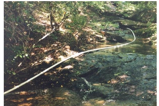
Figure 8. A PVC drive pipe placed in a stream bed. Galvanized steel was not an option due to the bed topography and geometry. The hydraulic ram pump worked well, but each bend allowed a tiny portion of the shock wave to dissipate. A straight, galvanized steel pipe would have captured a larger shock wave and provided more pressure. Image credit: W. Bryan Smith, Clemson University.
