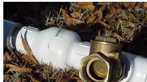
Figure 12. A brass swing check valve. Note the free-swinging flapper in the outlet port. The swing check valve should be placed vertically for best pump performance. Image credit: W. Bryan Smith, Clemson University.
