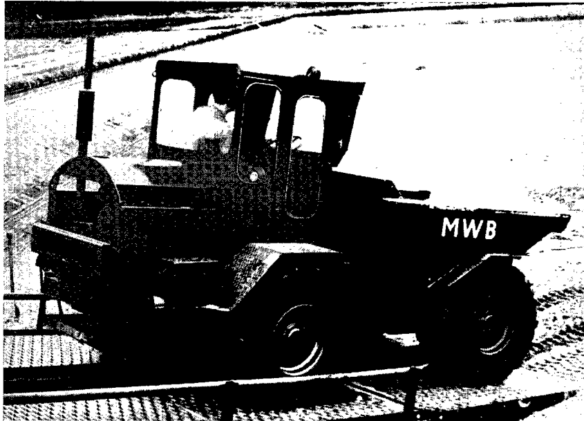
FIG. 34. FOUR-WHEEL-DRIVE DUMPER, 300 KG CAPACITY
