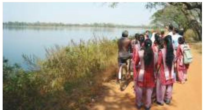
At a time when climate change is inducing more and more water scarcity in the region, restoring and conserving the traditional water harvesting structures such as Damodar Kata of Bijepur is of utmost importance.
