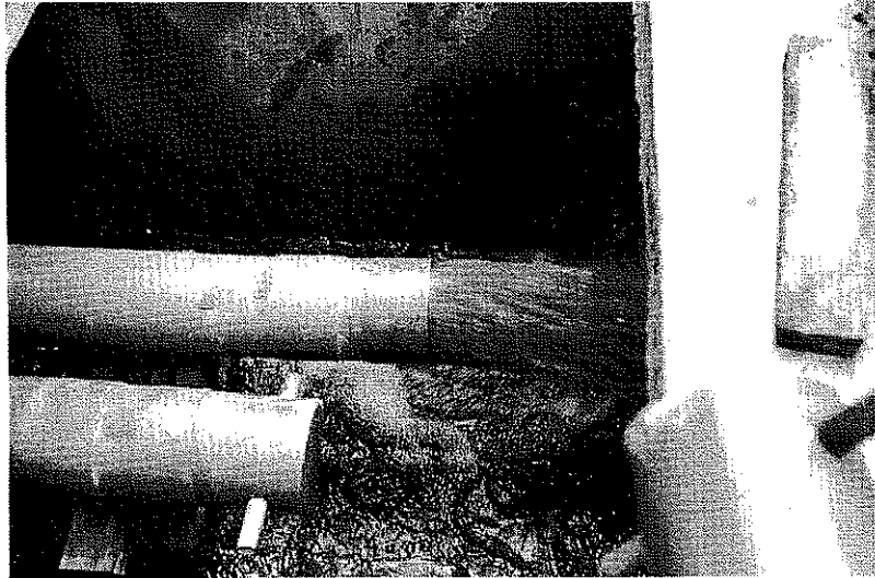
Photo 9 Hydraulic Cleaning of Roughing Filter (Note the Simple Design of the Fast Opening Device as also illustrated in Fig. 34, p. IX-9)
