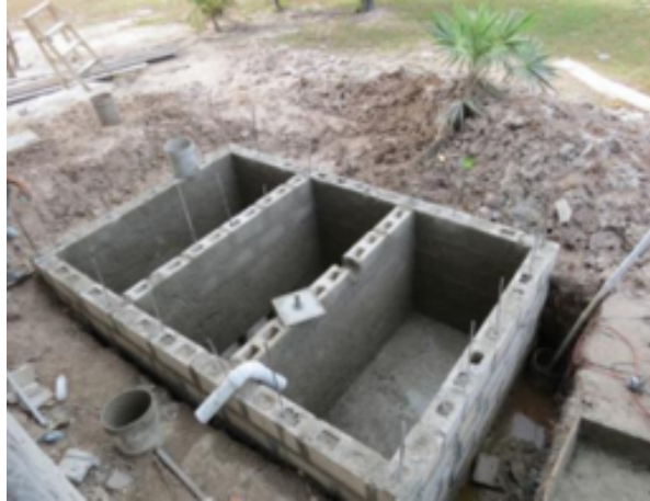
Figure 3: The Improved Septic Tank under Construction. Source: Sanitarios Jiménez.
