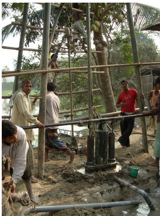
Fig. 9.6 Drilling a deep tubewell
