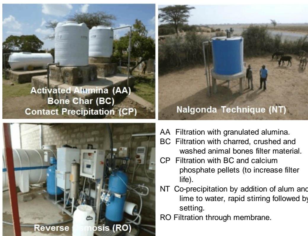
Fig. 9.9 Selected fluoride removal technologies
