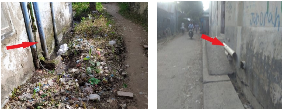
Figure 5: Containment technologies and their connections in Pabna. Left: Septic tank connected to nearby water body. Right: Toilet pipe connected to open drain.
