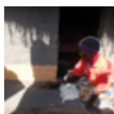
Rammed earth floor with small stones, sand, and smeared/polished 20
