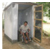
Latrine with level concrete entrance for wheelchair access 10
