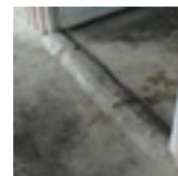
Slightly raised threshold to reduce flooding 11
