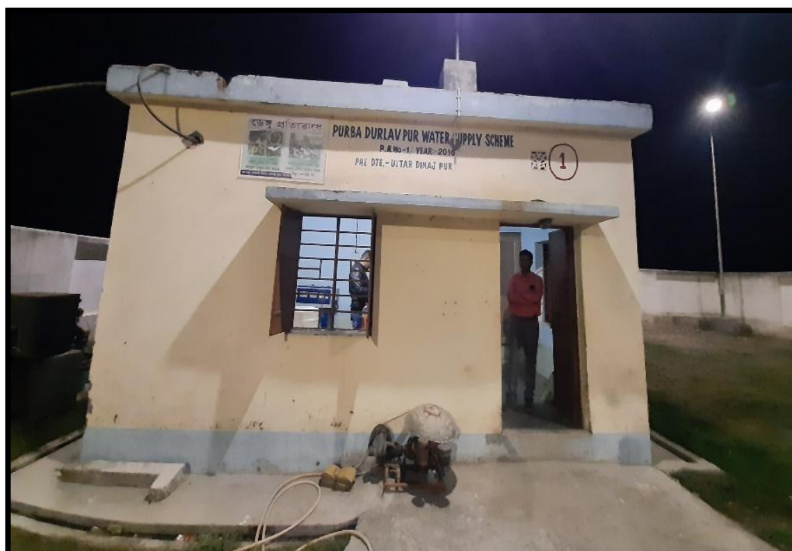
Image 8: Pump house at Purba Durlavpur Water Supply Scheme, Uttar Dinajpur
