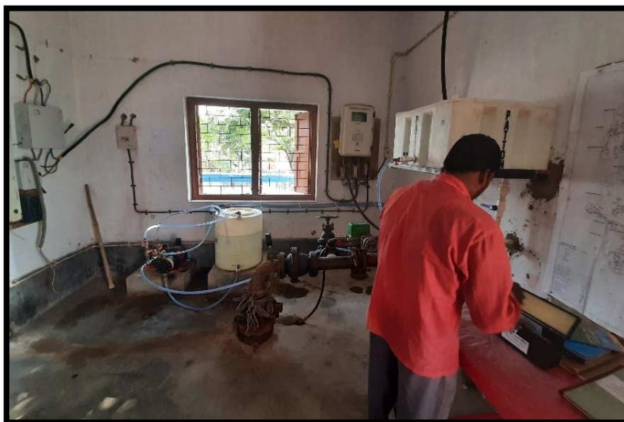
Image 2: Pump Operator measuring Free Residual Chlorine at pump house of Groundwater Based Water Supply Scheme for Gun Sankrul and Adjoining Mouzas, Malda
