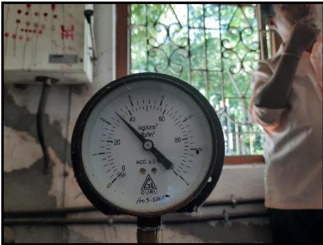
Image 3: Pressure gauge at pump house of Jateshwar Water Supply Scheme, Jalpaiguri
