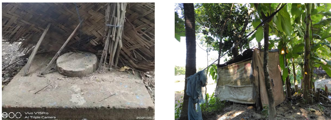
Figure 5: Septic tank and unimproved pit latrine in Lama.
