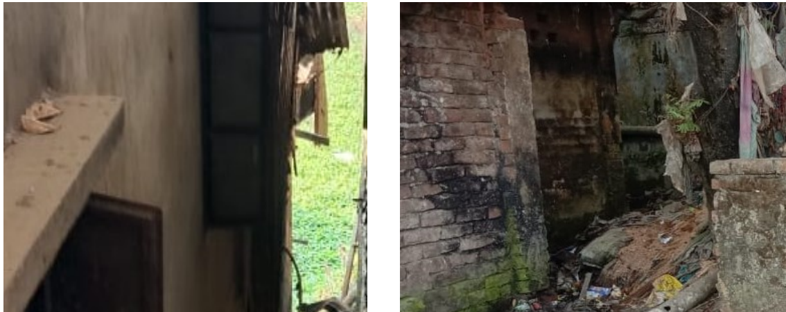
Figure 6: Containment technologies and their connections in Lama. Left: Septic tank connected to a nearby water body; Right: Toilet pipe connected to open drain.
