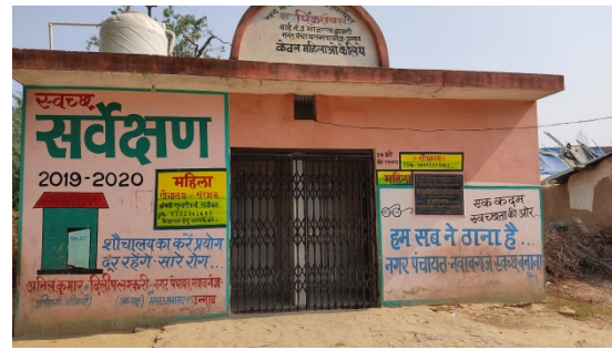
Figure 4: Pink toilet constructed under SBM.
