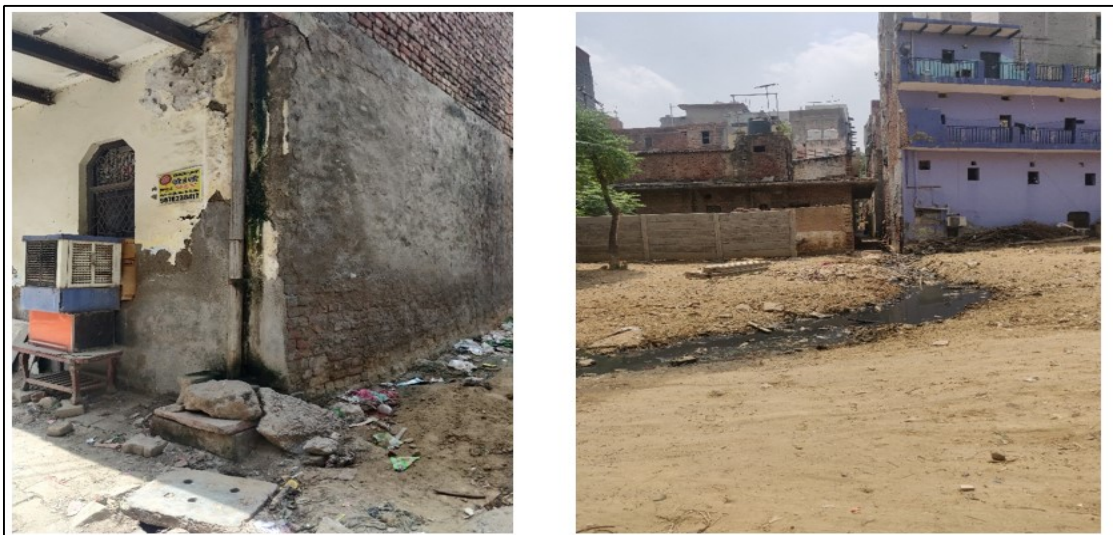
Figure 4: A toilet directly connected to underground sewer (left) and wastewater in kaccha drain before joining the drain (right) (Source: Uma/TRCSS, JNU (2021)).
