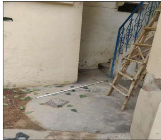
Figure 5: Lined tank with open bottom and impermeable walls in a household in Gurugram.
