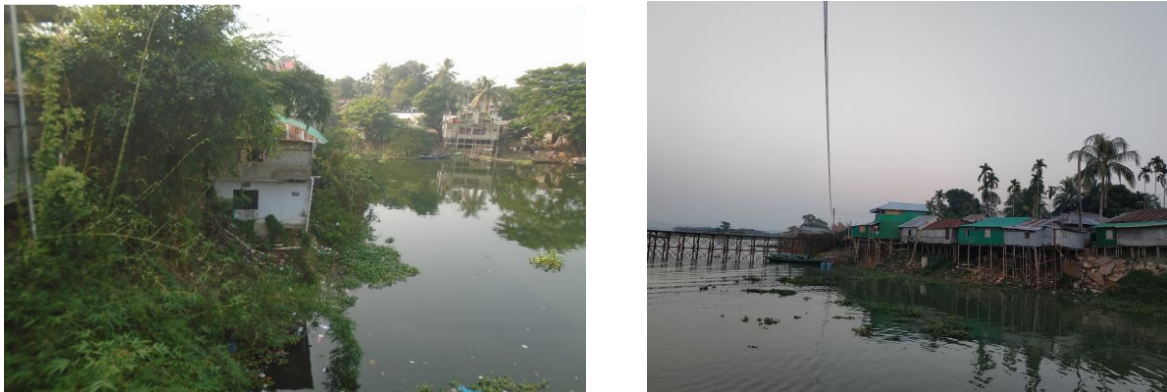
Figure 5: Toilet Pit and Pipe open to the Kaptai Lake, Rangamati.
