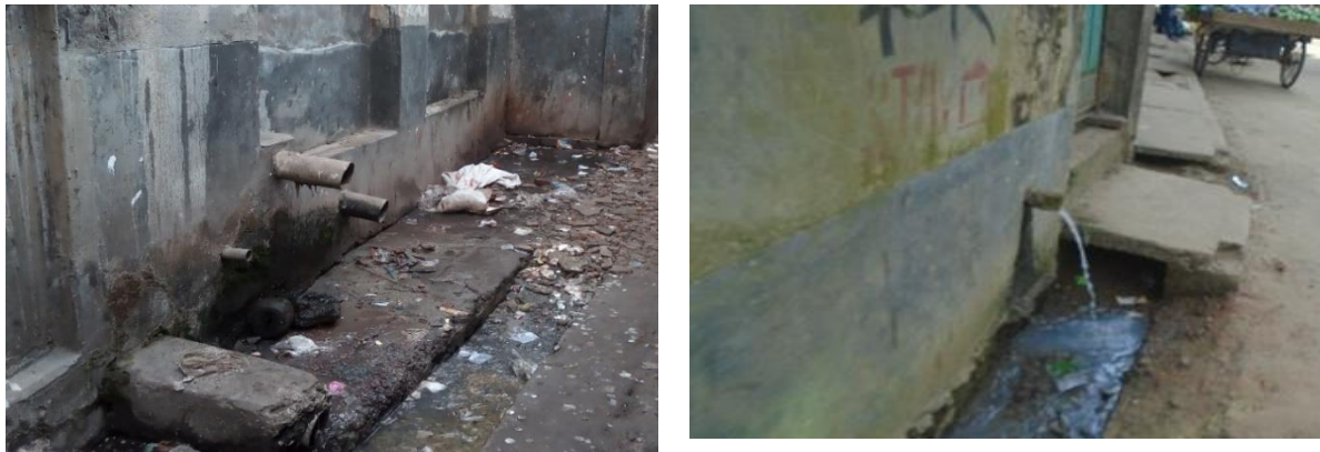
Figure 5: Containment technologies and their connections in Bandarban. Left: Septic tank connected to a nearby waterbody. Right: Toilet pipe connected to open drain
