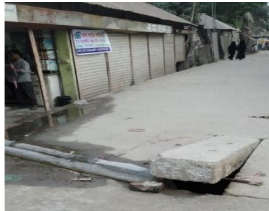
Right: Latrine delivery pipe connected with covered drain
