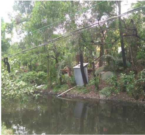
Left: Toilet Pit open to the nearby water body
