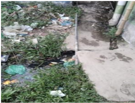
Left: Latrine delivery pipe connected with open drain
