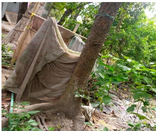
Left: Latrine delivery pipe connected with open ground
