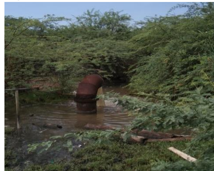
Figure 14: Sewage overflow pipe (Source: Gowtham/CSE/2021)
