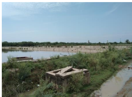
Figure 15: Water stabilization pond in Nathapettai STP (Source: Gowtham/CSE/2021)
