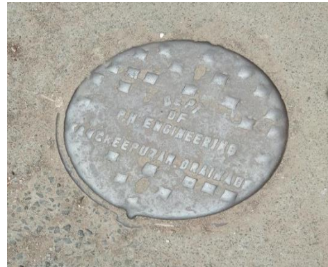
Figure 3: Drainage manhole cover in ward 21 (Source: Gowtham/CSE/2021)
