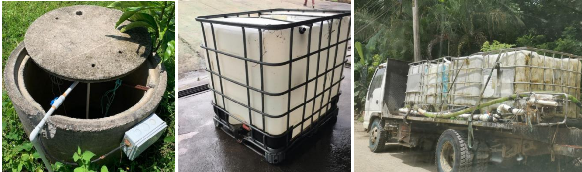
Figure 16: (Left) Example of a well drilled for domestic water supply; (Centre) Example of a water tank filled by trucks; (Right) Water delivery truck in Santa Teresa. Source: (Kenneth Alfaro Alvarado, 2021).
