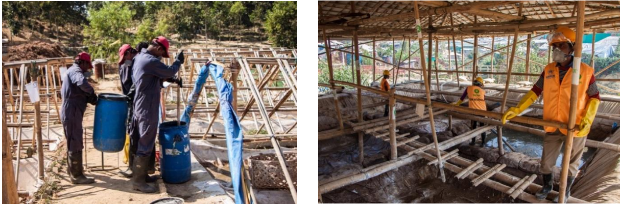
Figure 13: Example of Lime Treatment in a barrel. Right: Lime Treatment in Lagoon (Source: UPM, 2019).
