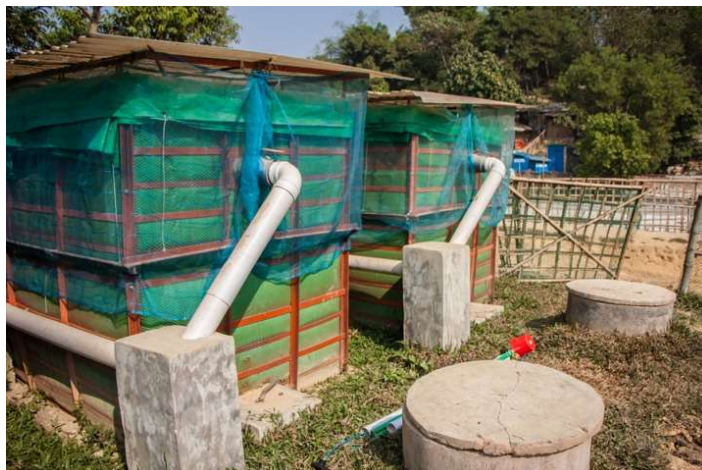
Figure 16: Anaerobic up-flow filter system (Source: UPM, 2019).
