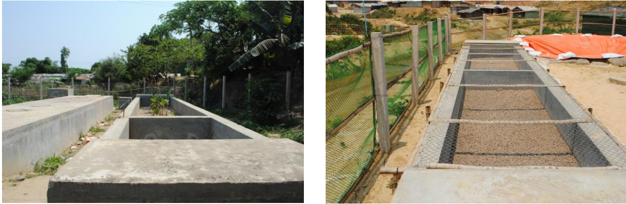
Figure 14: Example of Horizontal Constructed Wetland. Right: Horizontal Gravel Filter (Source: UPM 2019).
