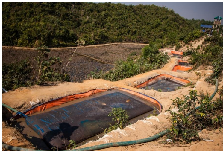
Figure 15: Example of Geo-Tube FSTP (Source: UPM, 2019).
