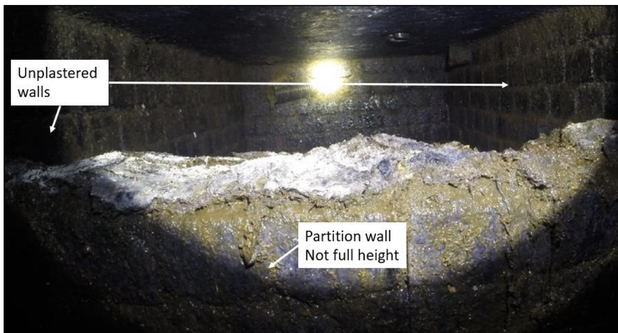
Figure 11: Lined pit with impermeable walls and open base, called a "holding tank" locally. (Source: Author, 2019)
