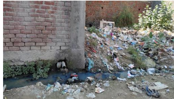
Figure 11: Fully lined tank connected to open ground, Zone 3 (Source: Urja Vashishth/CSE/2021).
