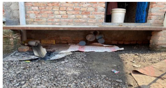
Figure 9: Fully lined tank with no outlet in Zone 2, Jaitpur Village (Source: Urja Vashishth/CSE/ 2021).
