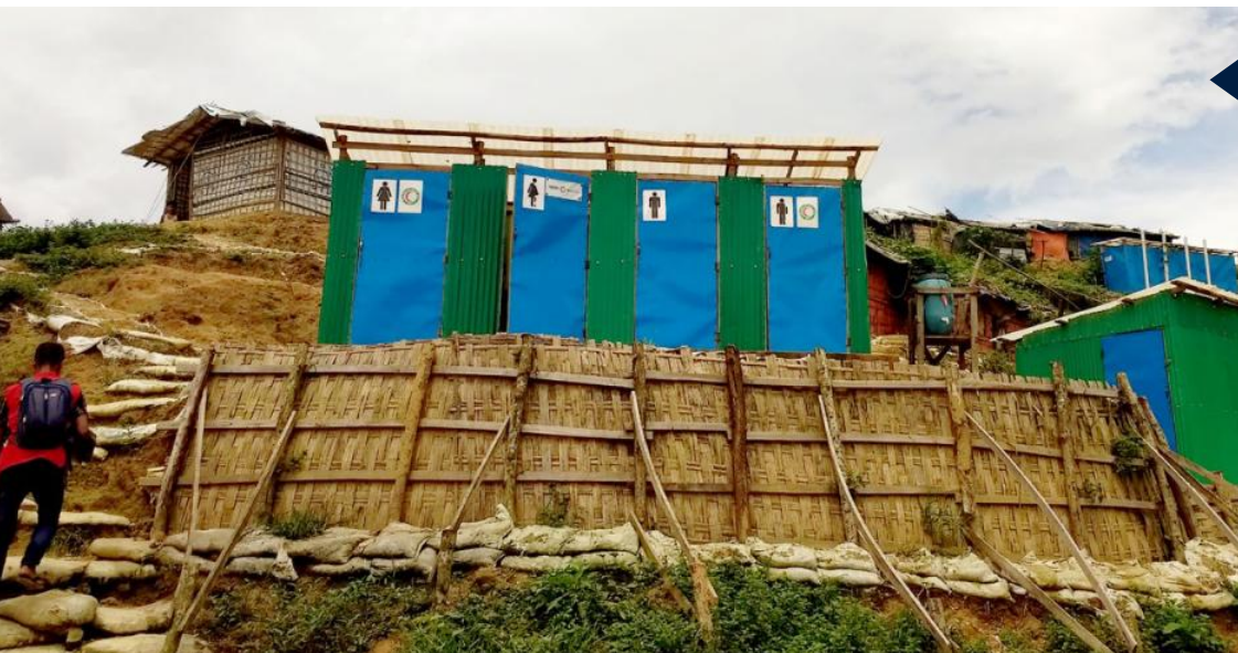
Block of latrines in Cox's Bazar
